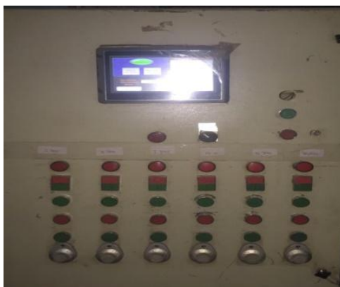
Figure 7 HMI with PLC
